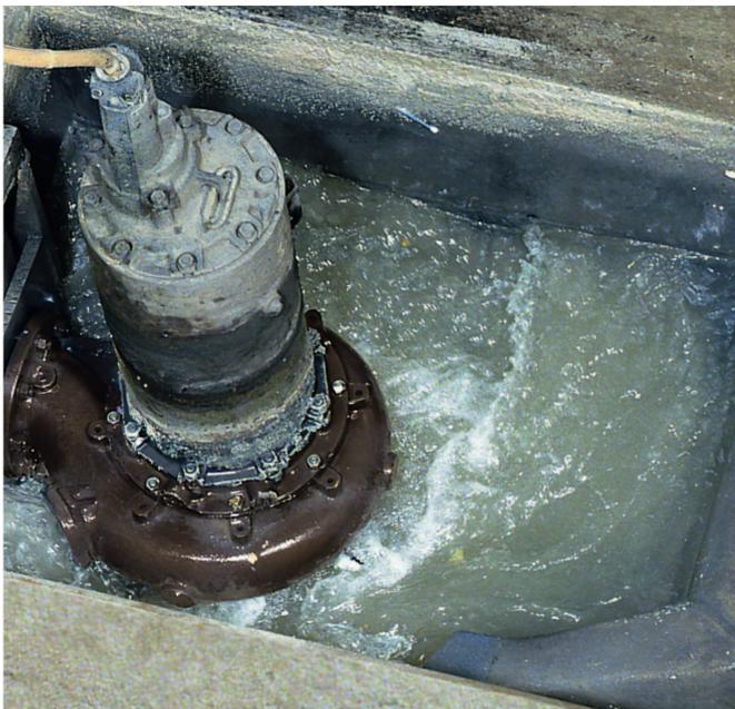
Sewage pump with immersible motor in wet well
